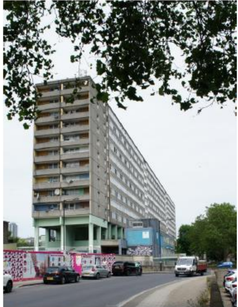
5. The full length of the facade is visible at the kink in Thurlow Street
