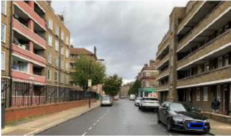
3. The existing LCC housing blocks along Kinglake Street
